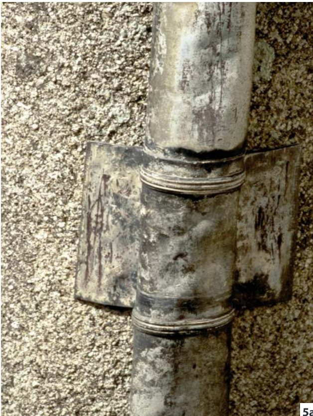
Figure 5: Collars: (a) Early 'false' collar and spigot joint formed simply by opening and closing the ends of the lower and upper pipes respectively, and applying cast astragals to the lower pipe, along with a band to create ears for fixing to the wall. (b) Typical plain collar fabricated separately as a wide cylinder, with cast astragals, and slipped over the lower pipe to form the collar to receive the spigot.
