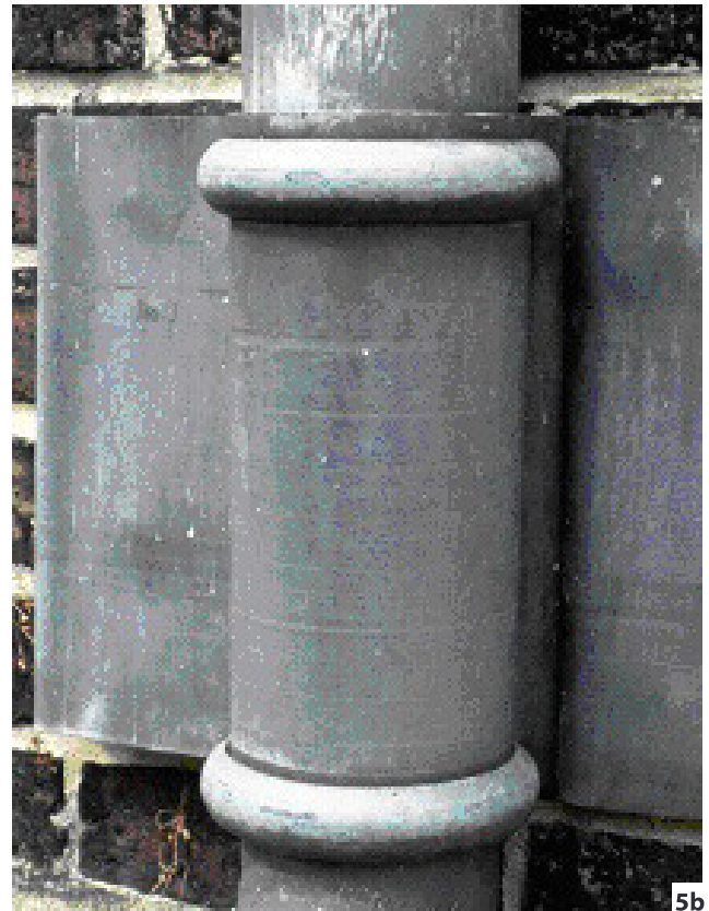
Figure 5: Collars: (a) Early 'false' collar and spigot joint formed simply by opening and closing the ends of the lower and upper pipes respectively, and applying cast astragals to the lower pipe, along with a band to create ears for fixing to the wall. (b) Typical plain collar fabricated separately as a wide cylinder, with cast astragals, and slipped over the lower pipe to form the collar to receive the spigot.
