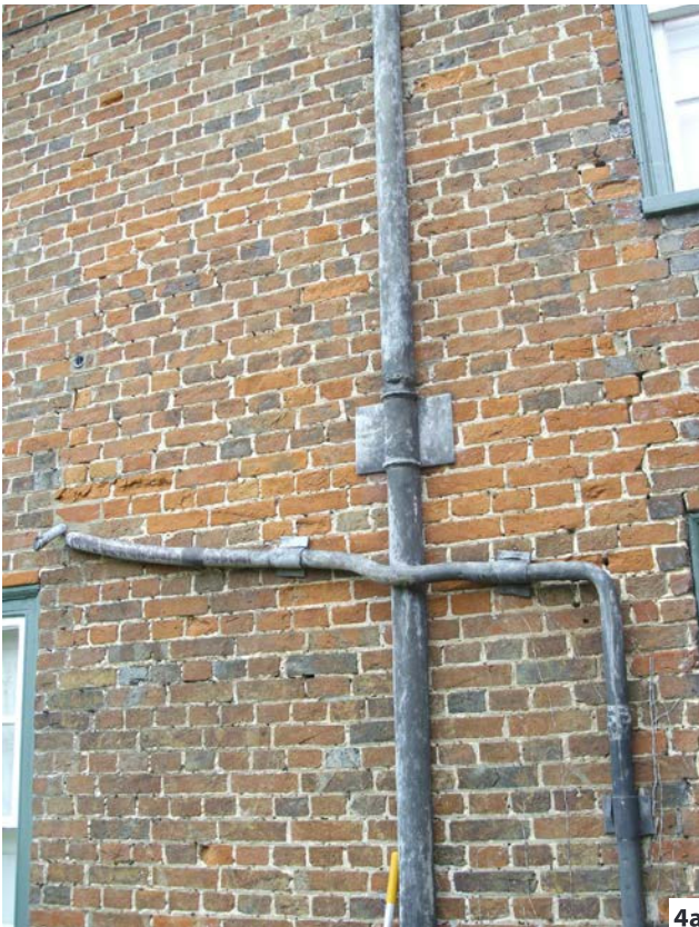
Figure 4: Lead drainage pipes: (a) Rainwater and waste water disposal. (b) For air venting, incorporating roof flashing. Photos: Douglas D Kent (a) and Peter T J Rumley (b)
