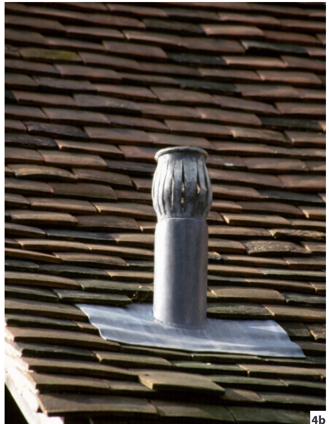
Figure 4: Lead drainage pipes: (a) Rainwater and waste water disposal. (b) For air venting, incorporating roof flashing. Photos: Douglas D Kent (a) and Peter T J Rumley (b)
