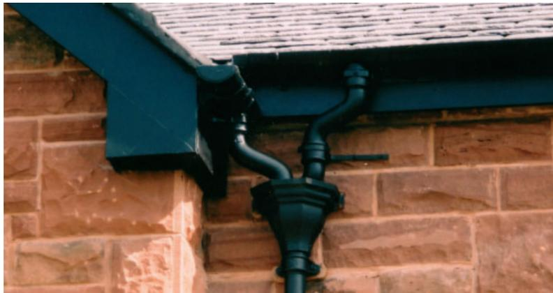
A reproduction of a typical late 19th century hopper with cast iron parapet gutters and simple ear bands on the down-pipe below
