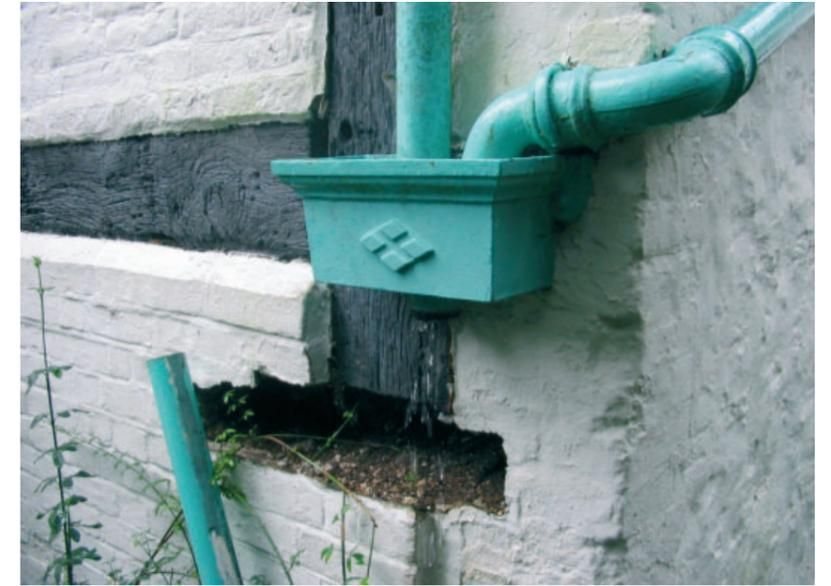
Without proper maintenance, damp and decay caused by blocked, sagging and damaged gutters can lead to expensive repair bills and the loss of historic fabric.
