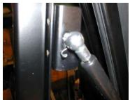
The brass winding mechanism is supplied for daily use of the window as we do not recommend using the gas struts for regular opening.
